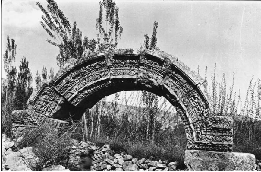
Fig. 2.6.4 Archway near basilica
